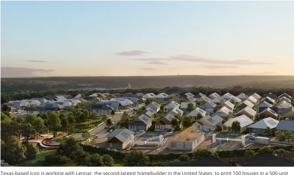
Texas-based Icon is working with Lennar, the second-largest homebuilder in the United States, to print 100 houses in a 500-unit development with architecture co-designed by Bjarke Ingels Group outside Austin. Lennar/Icon
